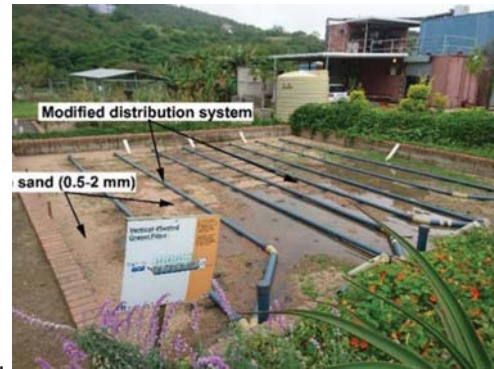
Appendix 6: Modifications to the demonstration-scale vertical flow constructed wetland. a. Redesign of the distribution system on the surface of the VFCW for even distribution of the wastewater; b. Temporal surface water accumulation after dosing to improve the retention time within the bed
