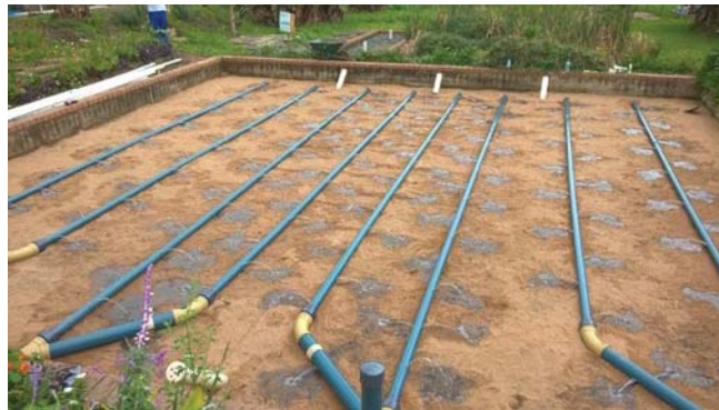
Appendix 6: Modifications to the demonstration-scale vertical flow constructed wetland. a. Redesign of the distribution system on the surface of the VFCW for even distribution of the wastewater; b. Temporal surface water accumulation after dosing to improve the retention time within the bed
