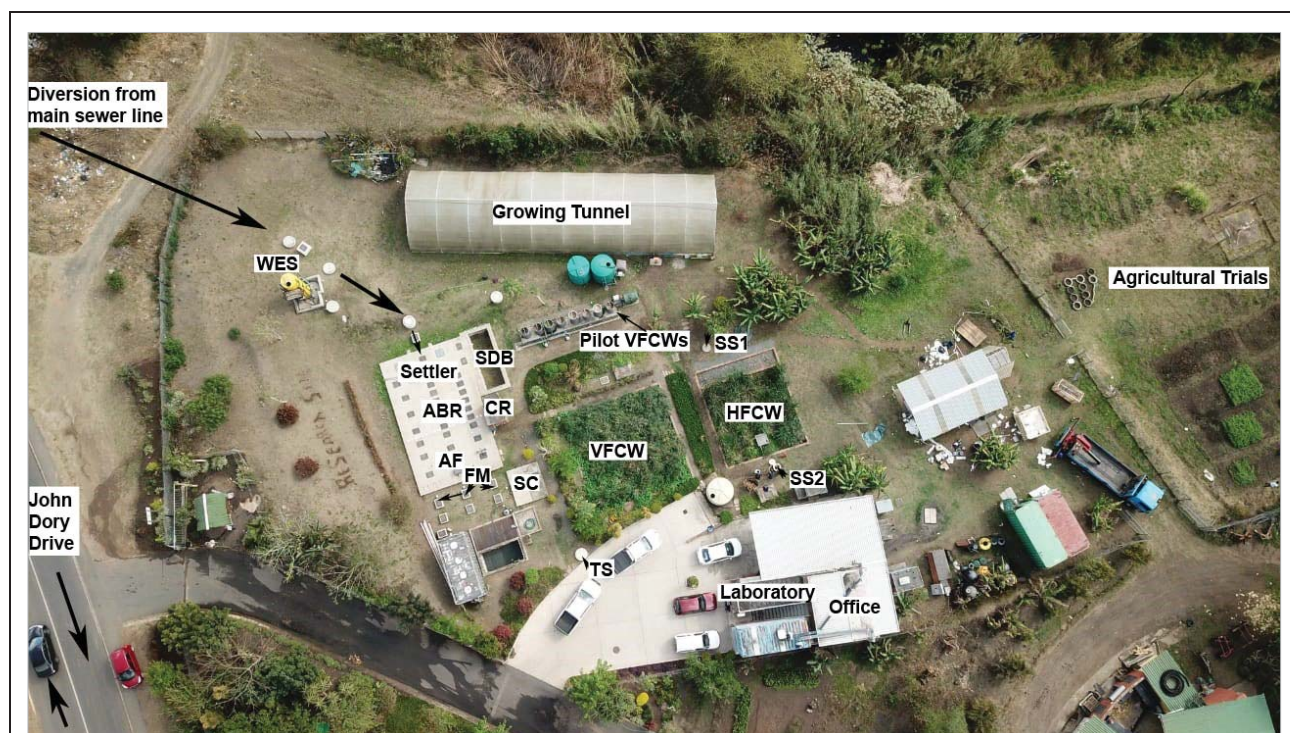
Figure 1: Aerial view of the Newlands Mashu decentralised wastewater treatment system, eThekweni (taken September 2019)
