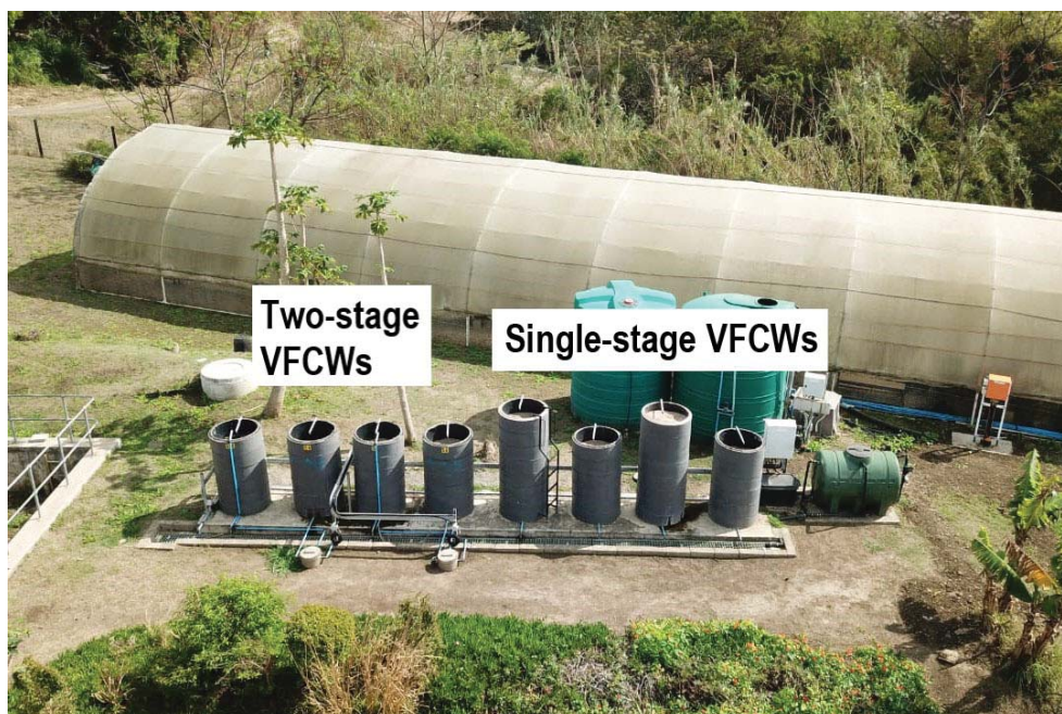
Figure 4: Pilot-scale vertical flow constructed wetlands treating anaerobically treated domestic effluent
