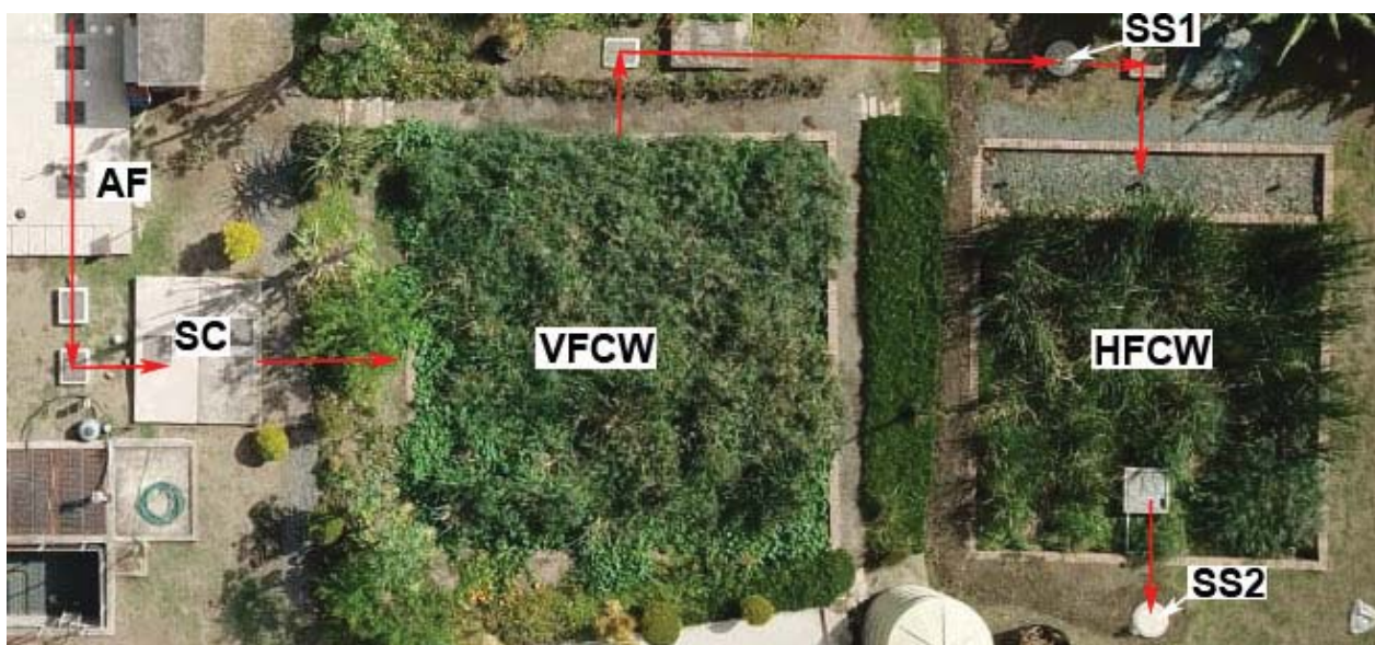
Figure 3: Aerial view of the hybrid sub-surface flow constructed wetland system (taken September 2019)
